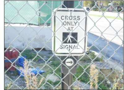
APS Device Behind Construction Fence
