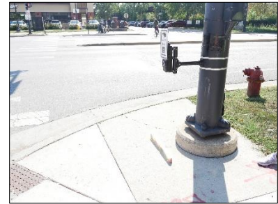
APS Assembly and Extension is a Protruding Object
