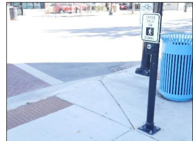
APS Placement at Typical 6' Curb Ramp
