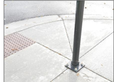
APS Pole in Curb Ramp Landing
