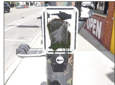
Vandalized APS Sign
