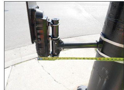
Object Protrudes > 12" from Pole or Foundation
